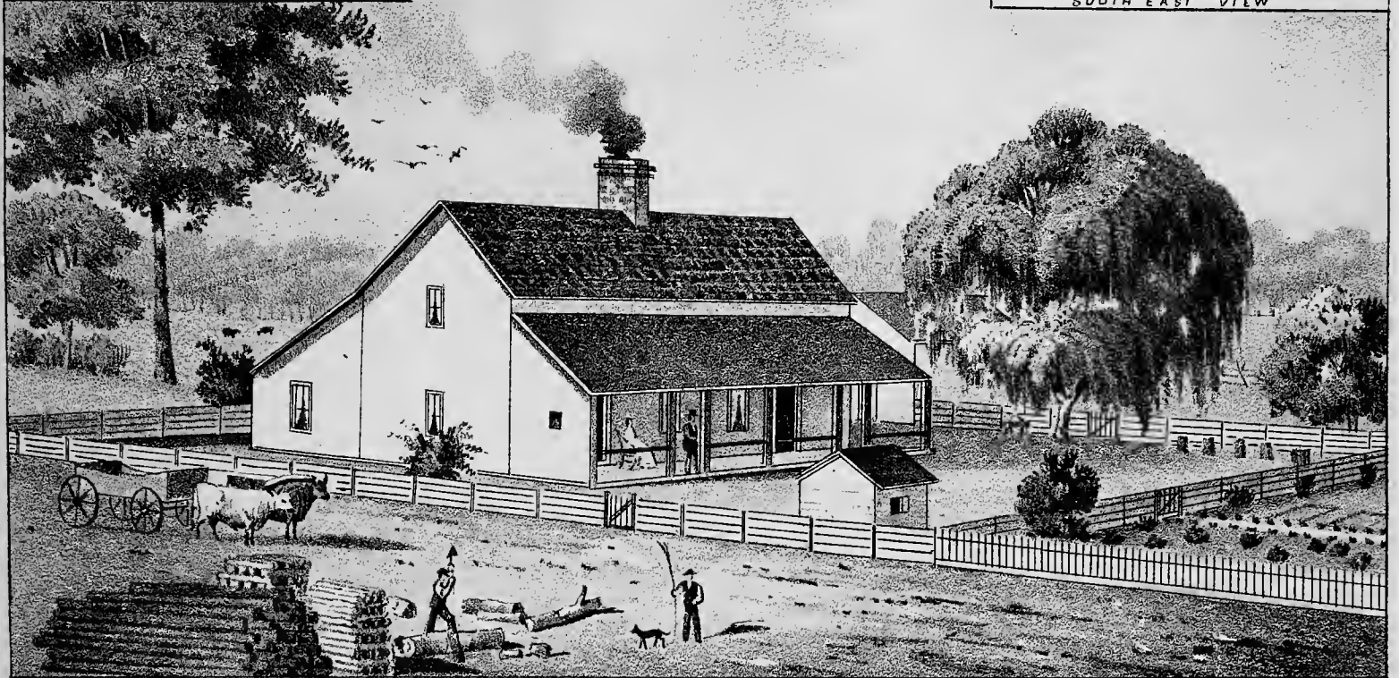
THE OLD STOOKEY HOMESTEAD IS REPRESENTED BY THE LOWER PICTURE, AS IT APPEARED FORTY YEARS AGO. THE HOUSE WAS BUILT IN 1802. THE VIEWS IN THE UPPER CORNERS SHOWS THE REMAINS OF THE OLD BUILDING AS IT NOW STANDS.
